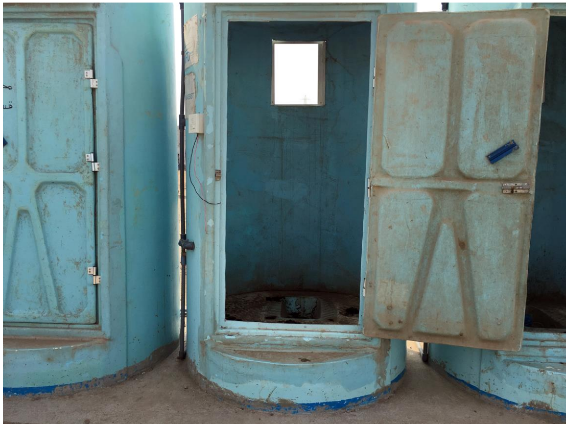
During a visit to Sabr Camp in Lahj, 12 June 2019, Amnesty International observed how latrines were inaccessible for persons with disabilities. These conditions, also observed in other camps visited by the organization, have an impact on persons with disabilities’ capacity to practise self-care and undermine their autonomy, privacy and inherent dignity. © Amnesty International
